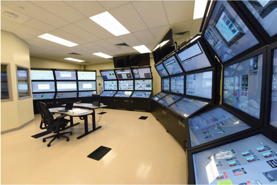
Fig. 1. The human systems simulation laboratory nuclear control room simulator. The hybrid COSS-CVCS is represented on the group of 3 bays depicted on the far left.
